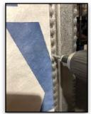
Repeat FM3 installation steps on one of the adjoining walls, making sure that the Vertical edge of FM3-VHV is flush with the edge/corner of the wall
